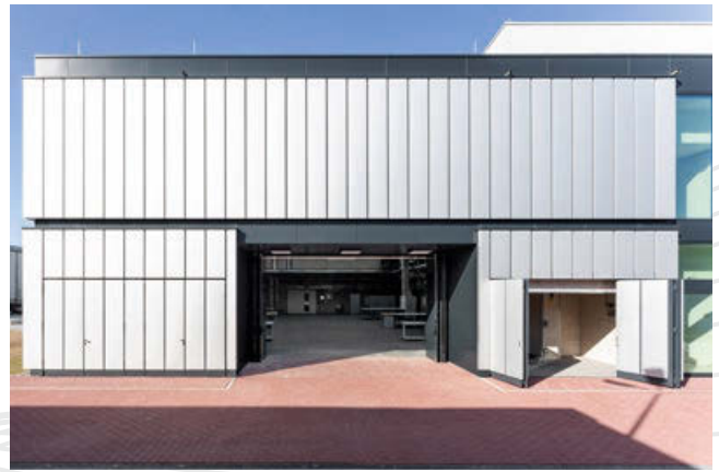
Rear view into the technical center
